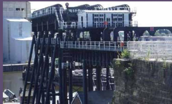
The completed lift was hailed as a great engineering triumph at the time but unfortunately it proved unreliable. The main problem was that hydraulic oil had not been discovered and so the fluid in the hydraulic system was water and, with all the salt around, the
