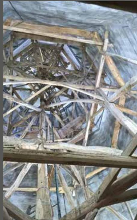
The photo in column 2 is taken looking up into the spire and shows the timbers in place which were used to construct the tower in the 13th century. These are still in use to the present day to provide access for repair and maintenance.
